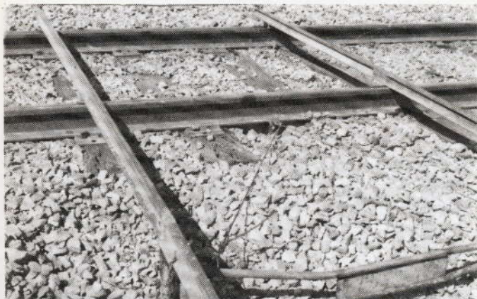
Anchor ropes and clamps attached to ensure stability and assist in maintaining the correct position in relation to the track.
